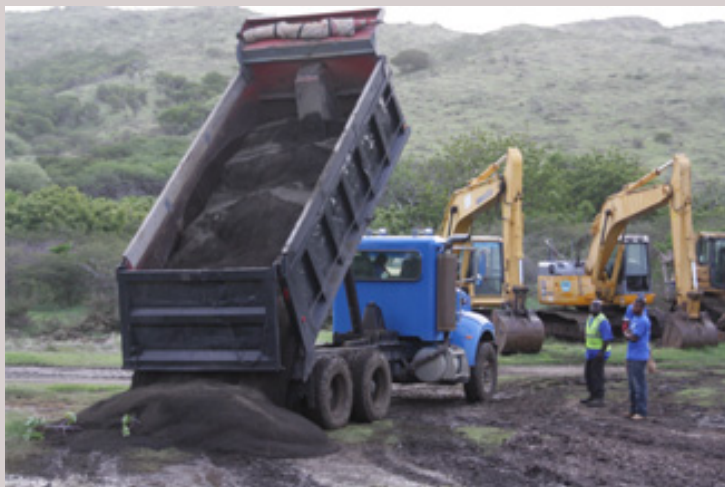
Work began immediately after the ground breaking ceremony on Monday afternoon.
